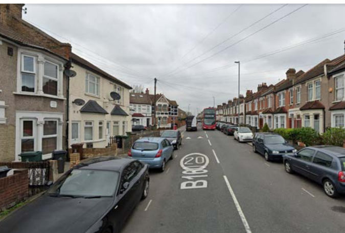
Key View 06: Winchester Road looking north
