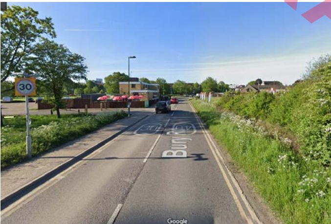
Key View 04: Bury Road looking south
