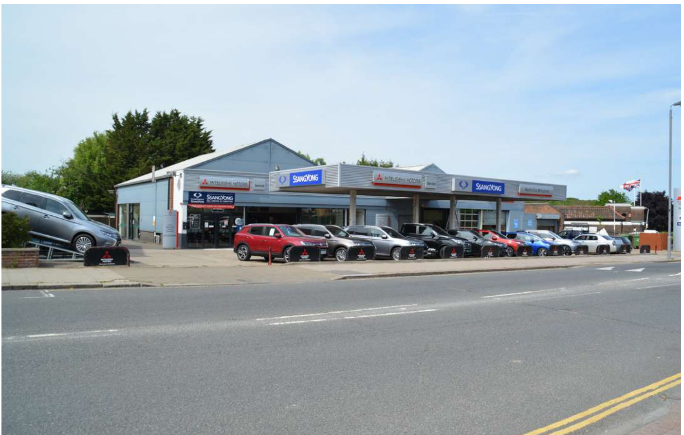
North City Motors, a major detractor at the gateway to Station Road.
