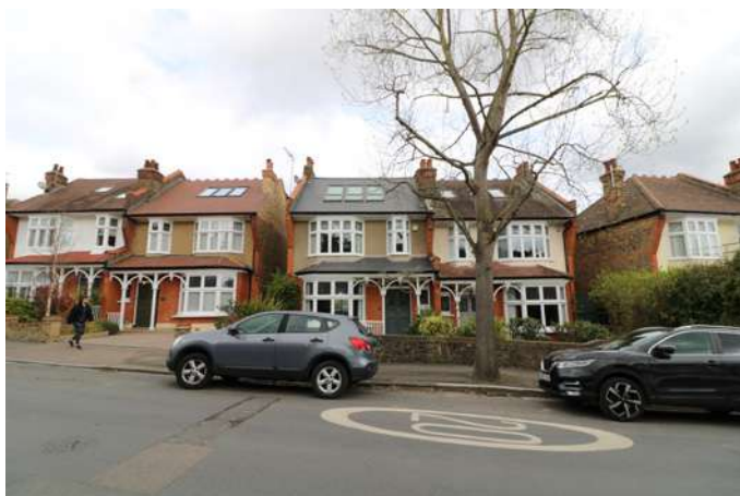
Rooflights to several Mornington Road properties
