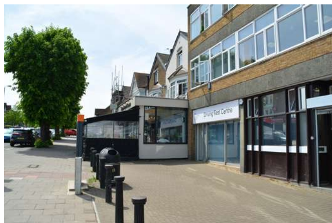
Encroachment on to pavements.
