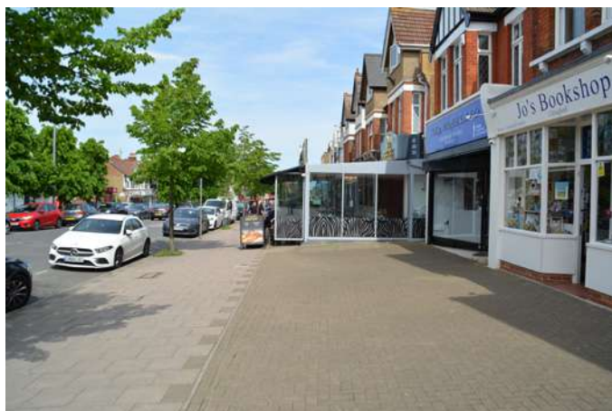
Encroachment on to pavements.
