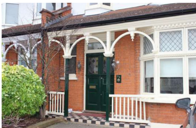
Good survival of timber porch with tiled flooring and original doors featuring leaded glass at 23 Gordon Road
