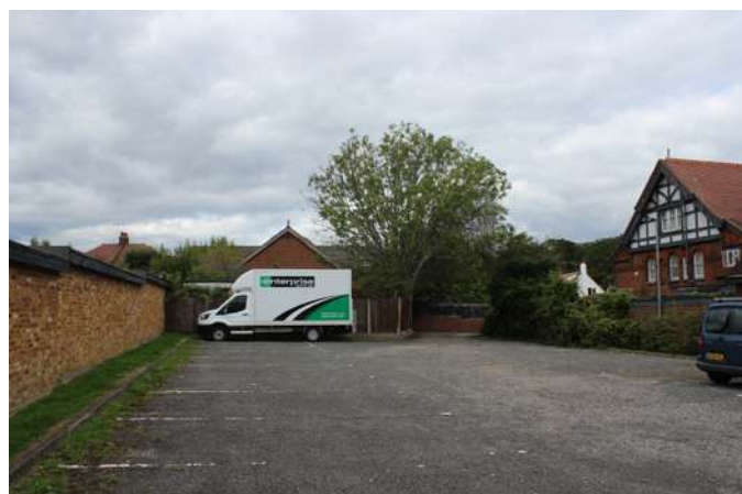
Poorly maintained tarmac hardstanding to the rear of the Queen Elizabeth Public House
