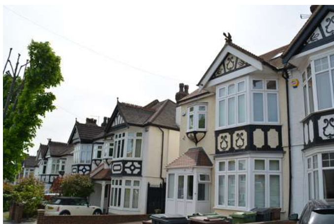
Two-storey villas on Beresford Road
