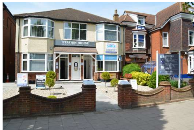
Extensive signage and sense of clutter.
