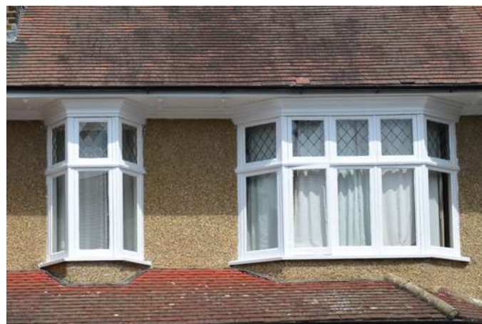
Original timber windows and stained glass.
