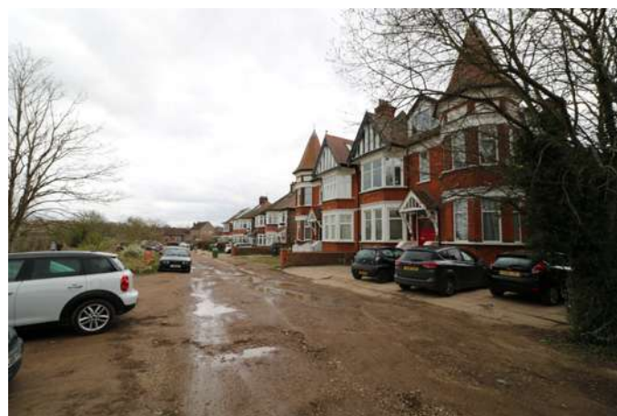
Loss of original boundary wall to accommodate off street parking.
