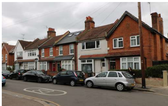
Loss of original windows and fenestration
