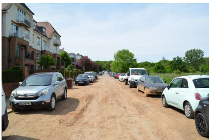
Substantial potholes along Forest View, a private unadopted road.
