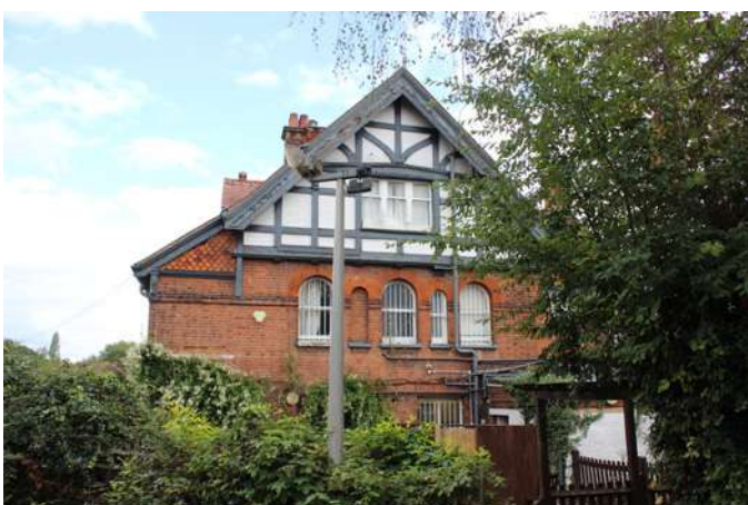
Rear (west) elevation of the Queen Elizabeth Public House which features exposed brick and hung tiling
