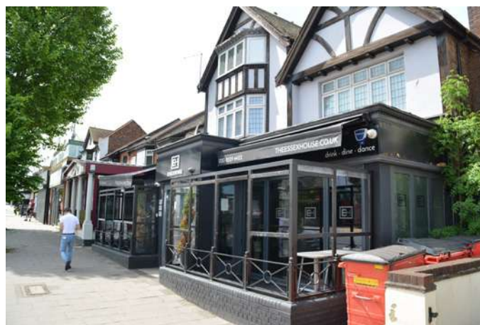
Loss of original frontage.
