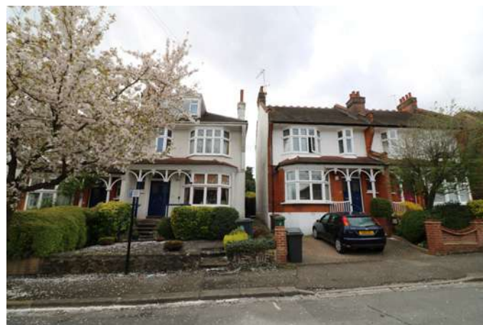
Loss of front gardens to off street parking
