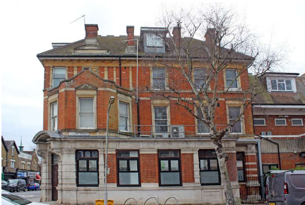
The former bank on the corner of Station Road and Willow Street comprising three storeys and attic level
