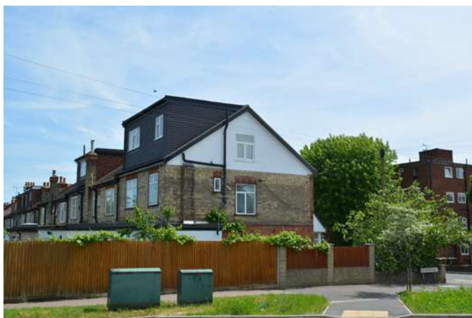
Bulky and visually intrusive roof extensions.
