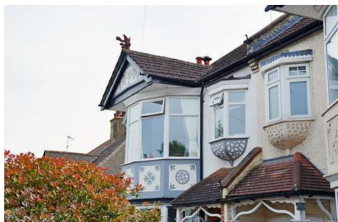
Decorative pargeting on Kimberley Road to gables, bay windows and oriel windows
