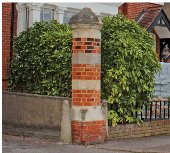
Historic brick and stone gate pier on Crescent Road
