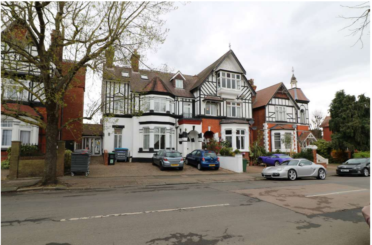
Loss of front boundary wall to off street parking.
