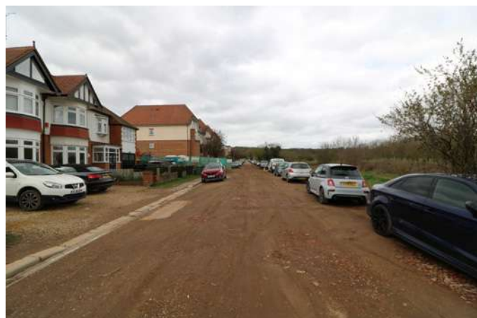
View looking west on Forest View.
