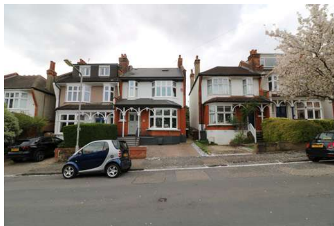
Unsympathetic roof extensions
