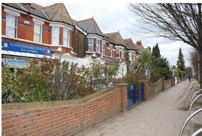
Leafy gardens at the west end of the character area (north side of the road)
