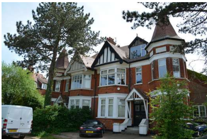
Dwelling boundary treatment removed to accommodate off-street parking
