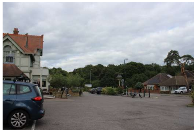
The large area of tarmac hardstanding in front of the Queen Elizabeth Public House, diluting the connection between the building and Whitehall Plain
